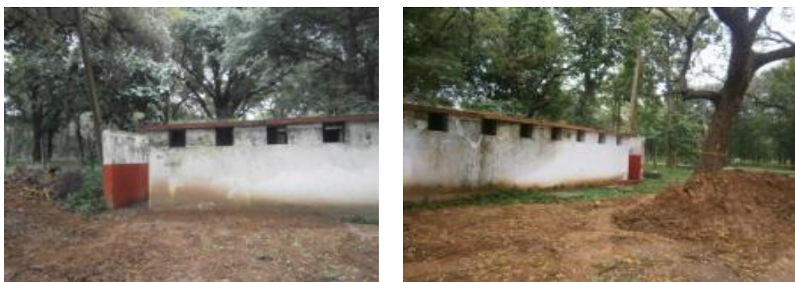
Figure 5.21. Public Toilet Rooms in Kataragama
